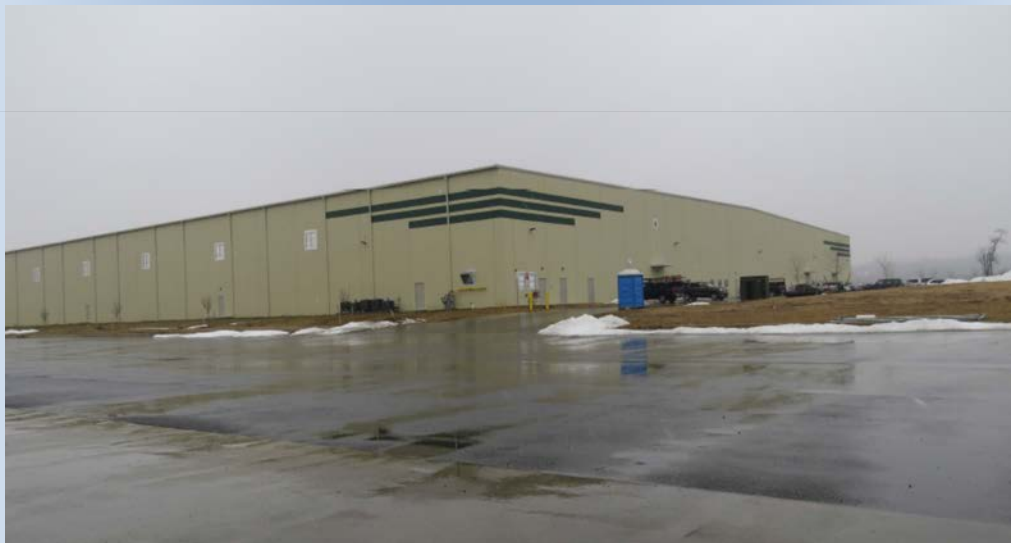
Trex project at Blackburn Commerce Center
