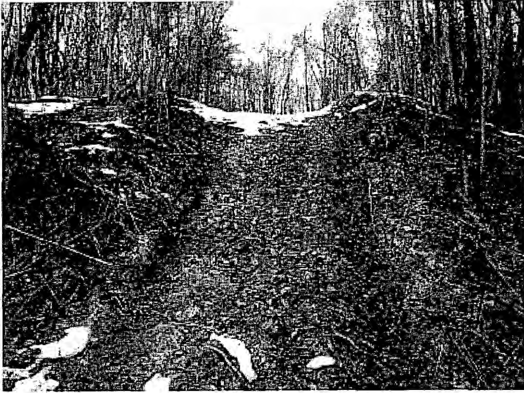
After ATV Scar Repaired by Mulched
