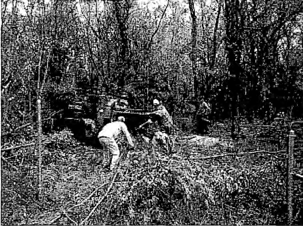
Before: Main gate during thinning
