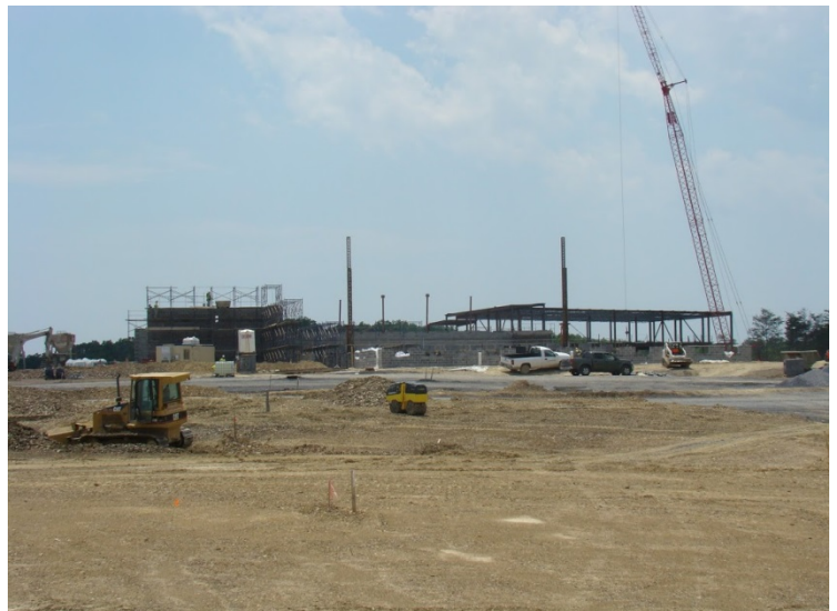
New Frederick County Middle School Construction
