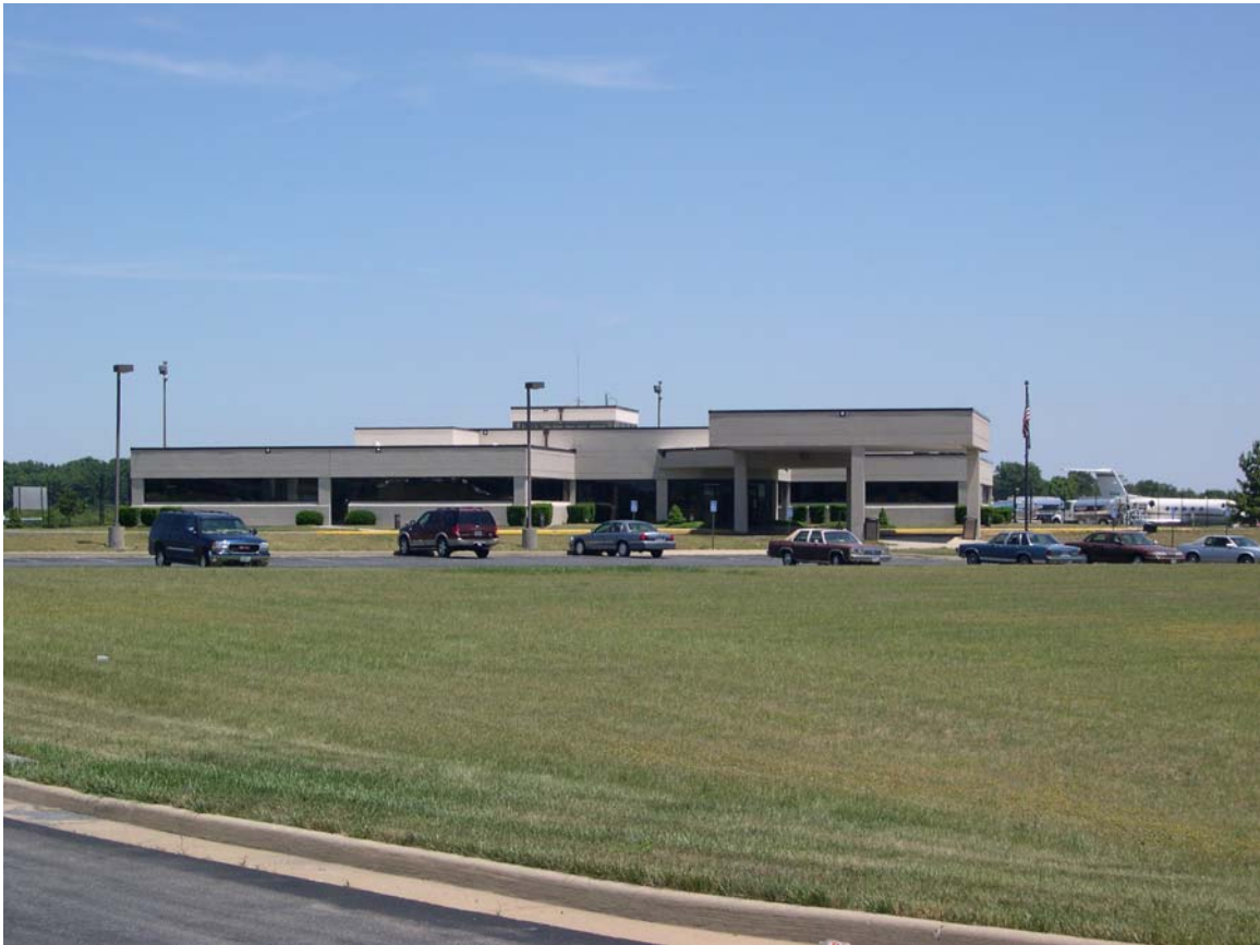
Winchester Regional Airport Winchester, Virginia Established 1987
