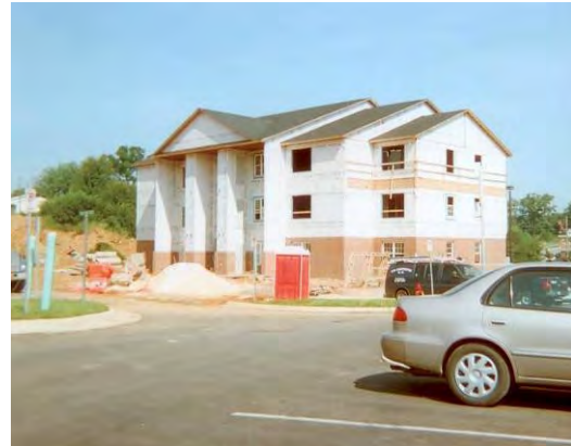
Building Under Construction
