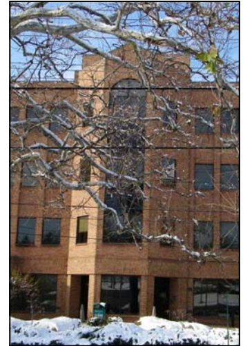
Photo courtesy of Lorraine Mossburg County Administration Building
