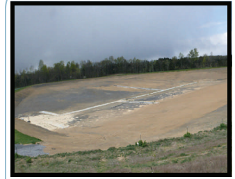
Construction Demolition Cell in Clarke County
