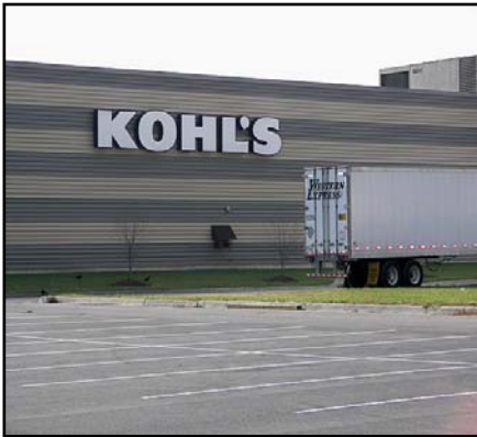
Kohl's Distribution Center
