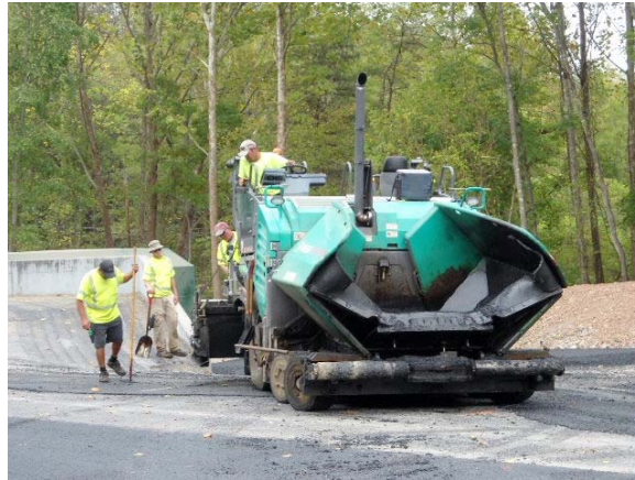
Paving underway at Round Hill Citizens Convenience site.
