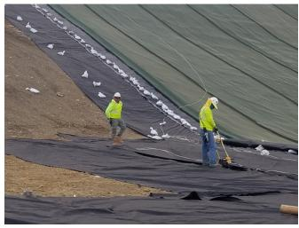
Temporary liner used as a "rain guard" being deployed to help decrease rain water infiltration, reducing the amount of leachate that is generated from the landfill.
