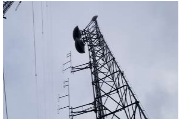
Figure 15: North Mountain Tower
