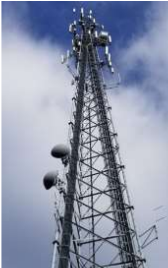
Figure 16: Brown Lane Tower
