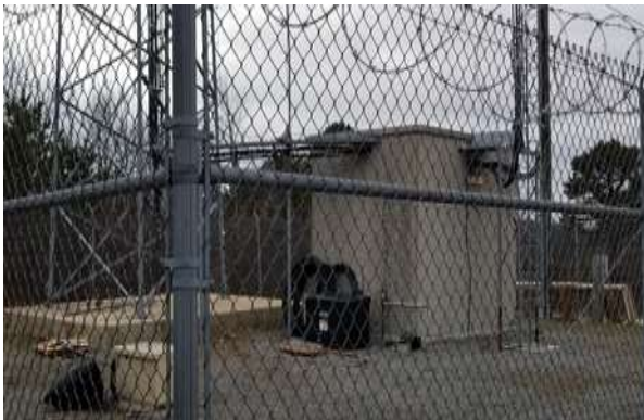
Figure 14: North Mountain Site
