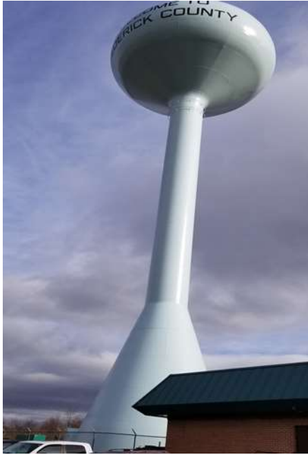
Figure 12: Tasker Water Tower
