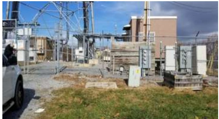
Figure 17: Brown Lane Site
