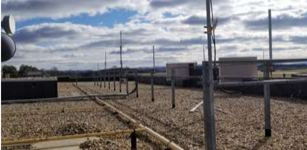
Figure 7: Frederick County Building roof
