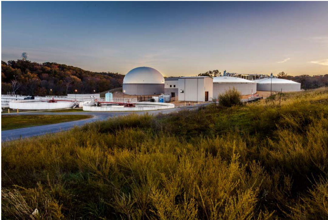
Green Energy Facility located at the Opequon Water Reclamation Facility on Route 7 in Frederick County.
